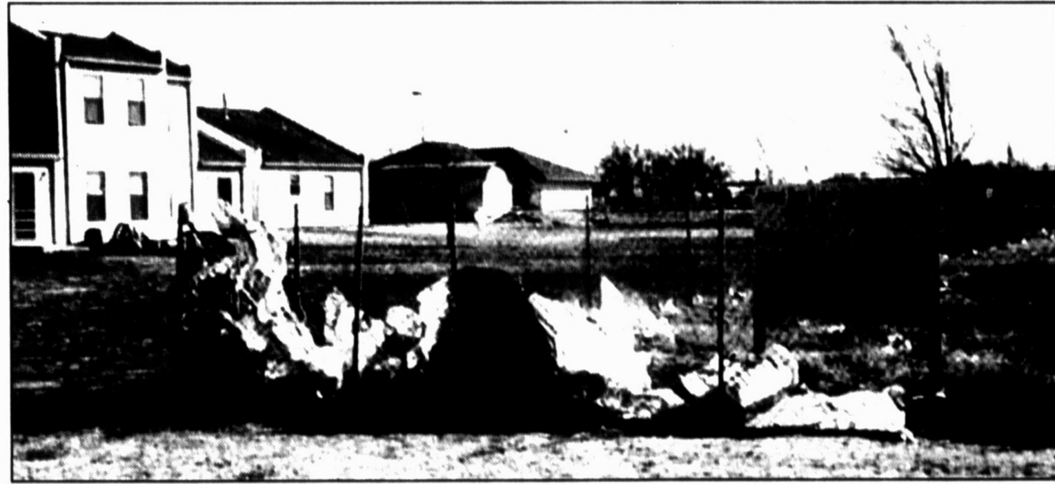
Trash-catcher? — The corner of a fence around the Amistad Farm Labor Housing construction site acted as a catcher for trash blown across the area Thursday afternoon by strong winds. The sustained winds hit 43 mph while gusts reached as high as 60 mph.
