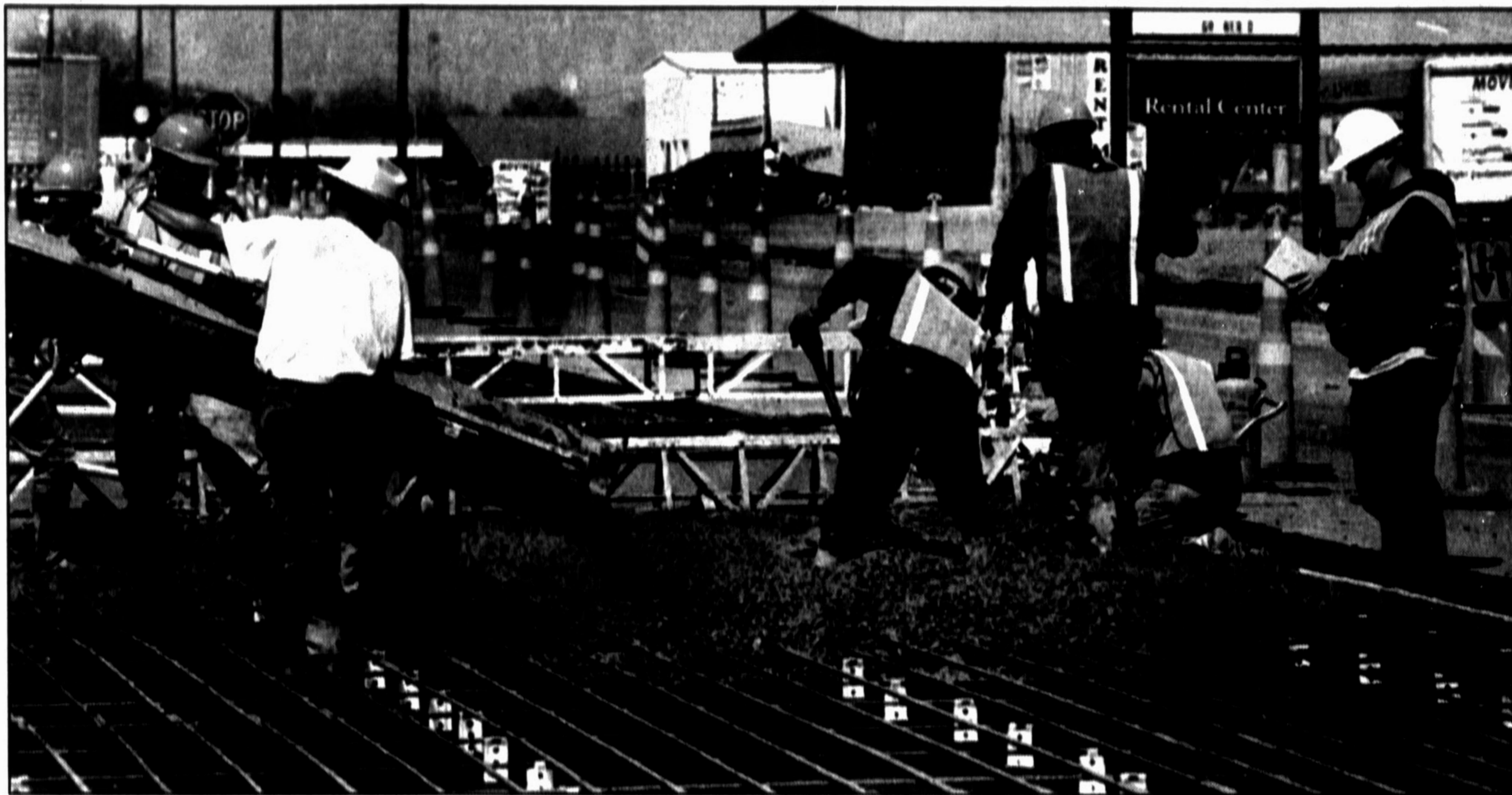
Pouring concrete — Workers with Pioneer Concrete of Hereford took advantage of a sunny day to pour concrete Wednesday at a section of U.S. Highway 385, just north of 15th Street. The state highway department is rehabilitating the roadway from the north city limits southward to U.S. Highway 60 (First Street). The construction project is expected to take about 15 months to complete.
