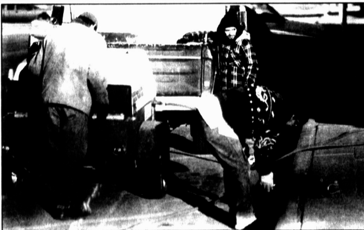
Replacing sidewalk — Patrons of the Hereford Post Office will have to use the south entrance for a few days while Gamez Concrete Co. workers replace the sidewalk in front of the building. Getting ready to break up the old sidewalk are (from left) Edward Bastardo, Lupe Ortiz and Al Gamez.
