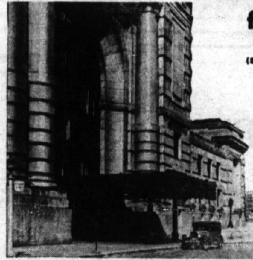
East entrance of Union Station, Kansas City
