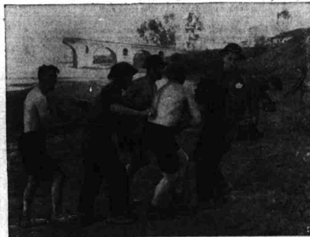
COMRADES CARRY WOUNDED SAPPER —A British engineer (sapper), wounded while repairing a bridge at Medjes El Bab, Tunisia, is carried up a river bank by his comrades.
