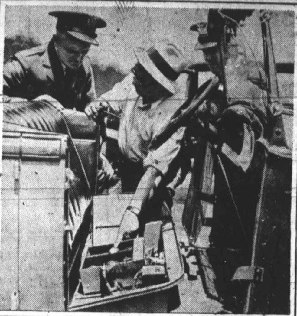
Installing a radio receiving set in a police car in Pasadena, Calif.
