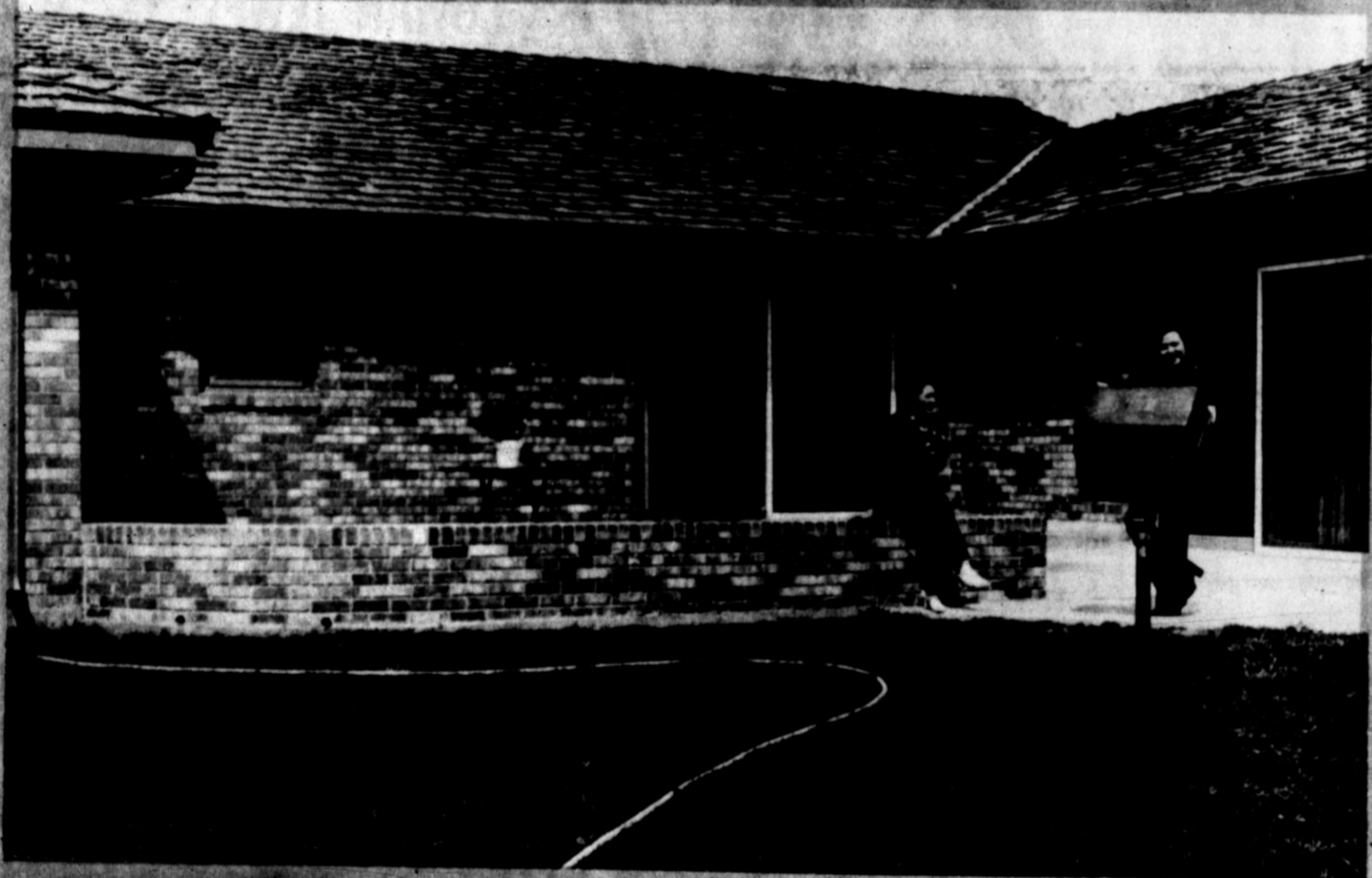
BUILT ANEW after it was struck by the tornado a year ago, the Earnest Langley home at 502 Star has a more attractive exterior as well as an interior replanned as a setting for the family activities. Between wings at the back where the storm demolished roof and walls, a wide patio is an ideal spot for outdoor meals and Mrs. Langley stands at a grill ready for cooking them. Mrs. Bruce Burney, a club hostess, is a visitor.
