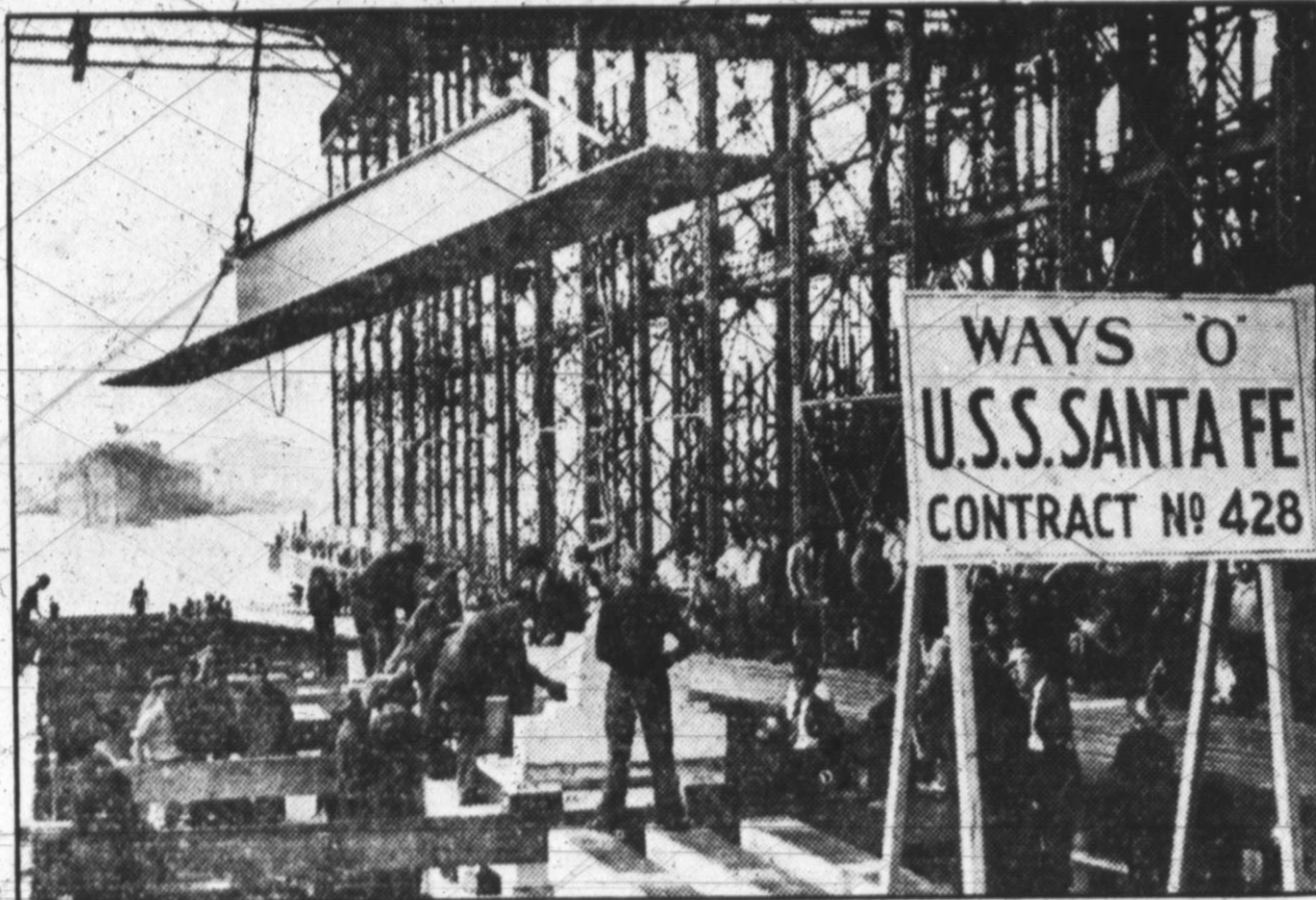
A minute after the U. S. S. South Dakota was launched, workmen began laying the keel for the 10,000-ton cruiser Santa Fe. In the background, the South Dakota, 35,000-ton battleship, sails the waters of the Delaware river. When she is commissioned, in less than a year, the Navy will have 18 of the 32 battleships needed for the two-ocean fleet.
