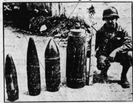
Sgt. William A. Hill of Charleston, S. C., holds measuring sticks beside four German shells of the type the Yanks are dodging on the Anzio beachhead. Left to right: 150-mm., 180-mm., 210-mm., 280-mm. (The "280" is minus its nosecap; all there, it would be about two feet longer.)
