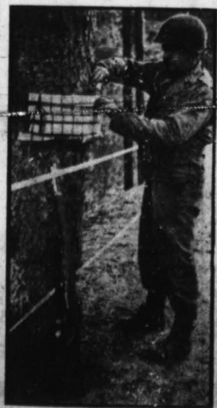
Pvt. John B. Brady of Philadelphia, Pa., and the 200th combat engineer battalion puts a charge around a tree in a defensive position near Bouillonville, Belgium. The explosives are placed in such a way that when set off the tree will fall across the road. (Signal Corps photo.)
