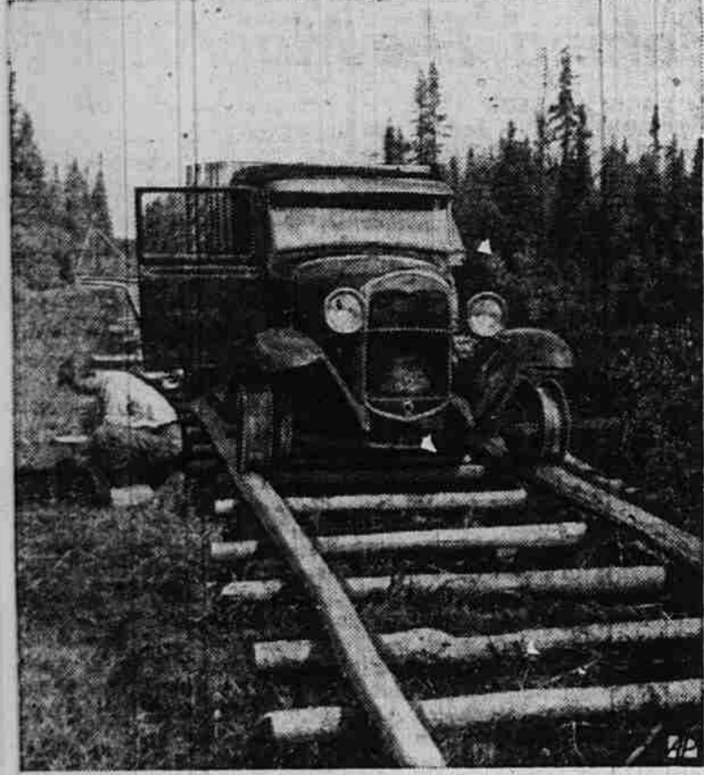
WATER FOR ENGINE —The "engine" on the Bour-lamaque Central railroad, built of saplings to reach seven miles across deep swamps in a new gold strike region of western Quebec, pauses to dip swamp water for his engine.
