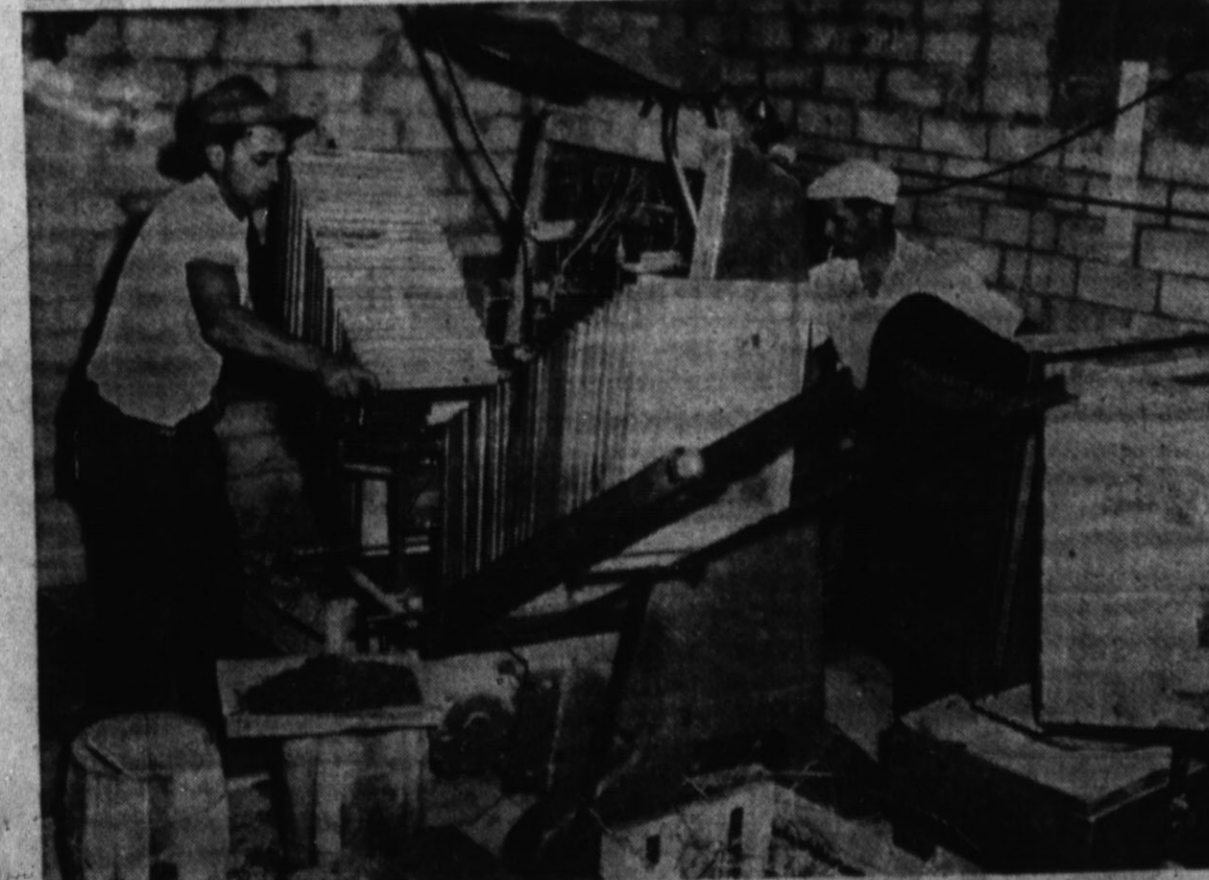
THERE'S NO END to the number of boxes that Charles Huston Co., produce shippers here will need when the company starts cutting and boxing for shipment Friday morning of the 1952 lettuce crop. The plant will
