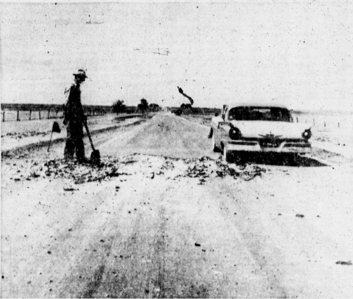
SUBMERGED since June 17, a section of U. S. 385 four miles north of Hereford was opened to through traffic Sunday afternoon this week. Unusually heavy rains this year left a temporary lake across the section for six weeks and two days. Repairs on the highway began immediately after the water level dropped below the highway surface. Motorists are warned to drive through the section under repair with extra caution. (Staff Photo)
