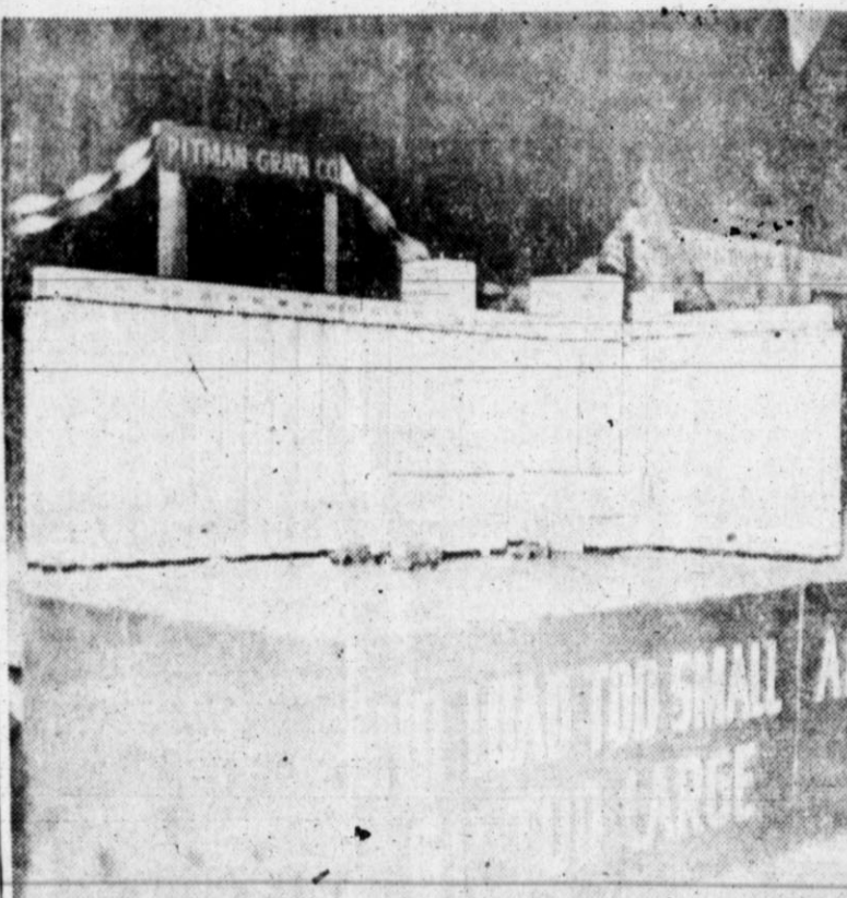
Pitman Grain Co. elevator (Staff Photo)
