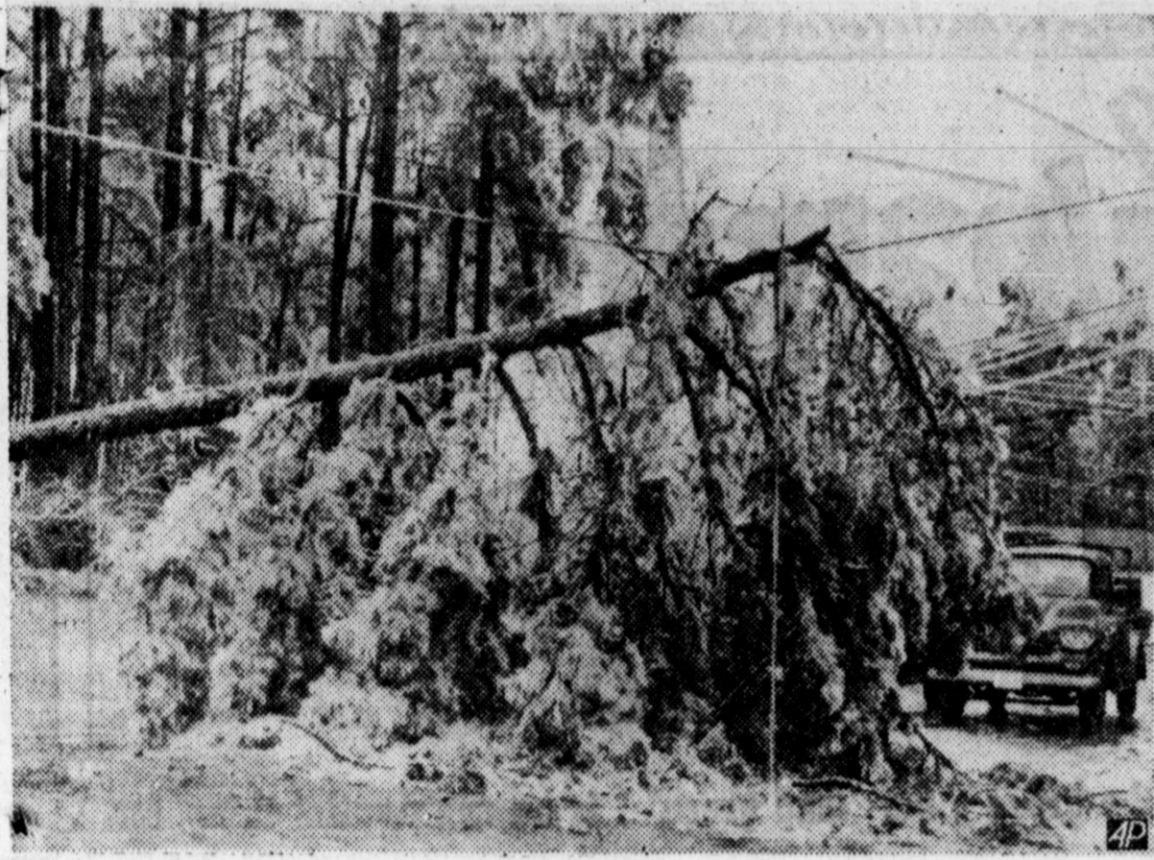
ICE STORM HITS HARD — A giant pine tree rests on a power line in Marshall, after a crippling ice storm struck the area causing trees to topple under the weight of the ice. Utility crews worked around the clock in sub-freezing weather in an effort to repair the damaged lines and restore power to homes. (AP Wirephoto)
