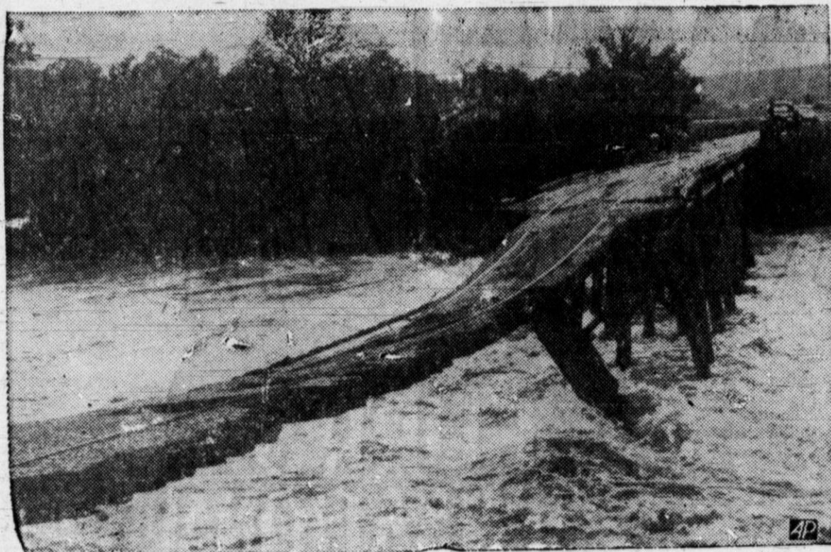
ALMOST GONE—Flood waters rushing over the spillway of Lake Texoma into Shawnee Creek near Denison washed out most of this railroad trestle. The trestle is on a spur track leading from the Denison Dam powerhouse to Yellow Jacket Boat Co., Inc. Engineers expected the bridge to give way. (AP Photo)
