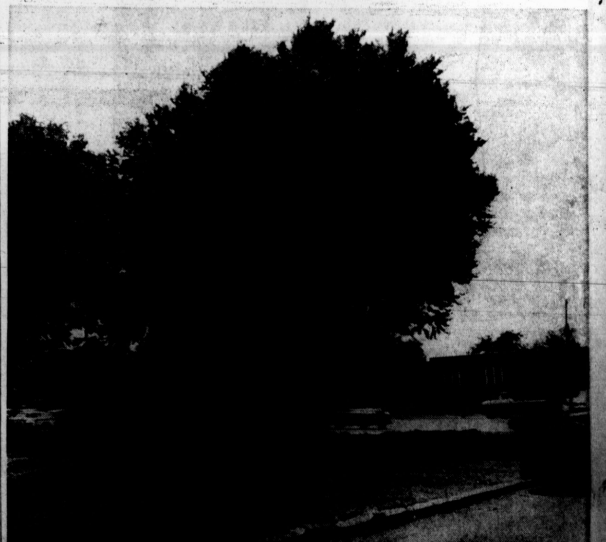
TIM-BER-R.—County Courthouse renovation operations were marked Tuesday by the absence of two trees fallen by J. W. Messer & Co. at the north side of the courthouse. Two powerful bulldozers and a laboring wench truck were required to uproot the stubborn 50 year old-plus elm. One of the trees is shown about one second before it thundered to the earth. (Staff Photo)
