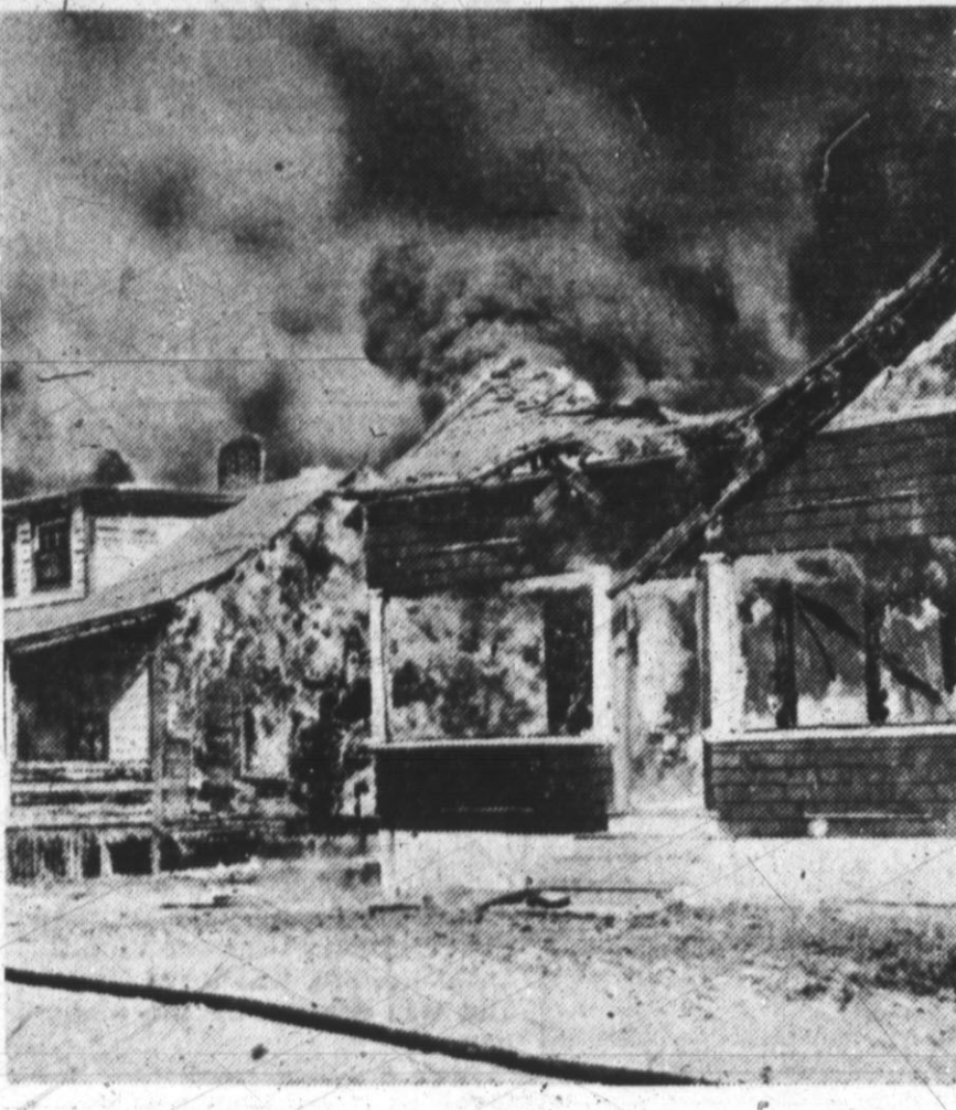
Damage estimated at about $2,000,000 was caused in the Ocean Bluffs, Mass., area as the result of a fire that destroyed a church and leveled more than 450 cottages. Only a timely shift in wind saved hundreds of other houses. The above photo shows a row of cottages burning fiercely when the fire was at its height.
