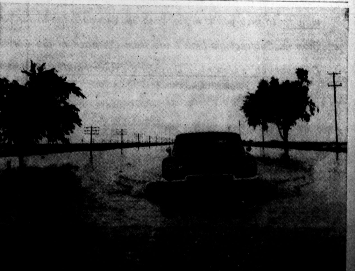
TRAFFIC WAS SLOW and hazardous on U. S. 60 Highway 60 east of Hereford Friday as a result of torrential rains. Small stakes at the edges of the paving provided the only guides for soggy cars that went creeping through three miles of water between Hereford and Dawn. Many motorists had to be pulled through by Texas Highway Department trucks. (Staff Photo)
