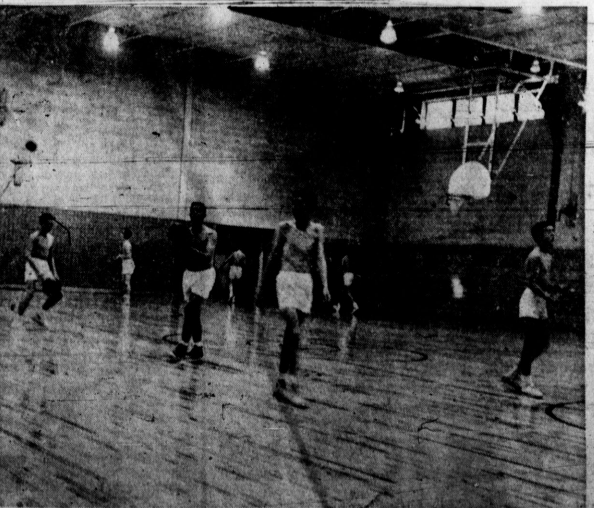
NEW GYMNASIUM for Stanton Junior High was used for the first time Monday. The large athletic facility is located in the same building as new classrooms. The main playing court is 50 feet by 80 feet, with four additional goals on the sides. Folding bleachers, at right, are installed on one side of the gym and will seat about 600. (Staff Photo)
