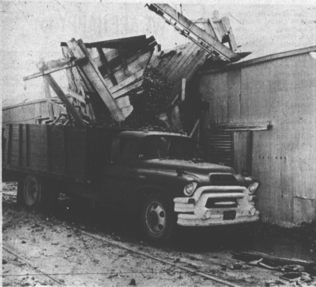
EXTENSIVE DAMAGE — 10,000 pounds of standing in the bin from the recent rains cull potatoes fell from this cull-bin at the Al Trautmann sheds, into the truck below causing extensive damage to the bin. Water Photo)
