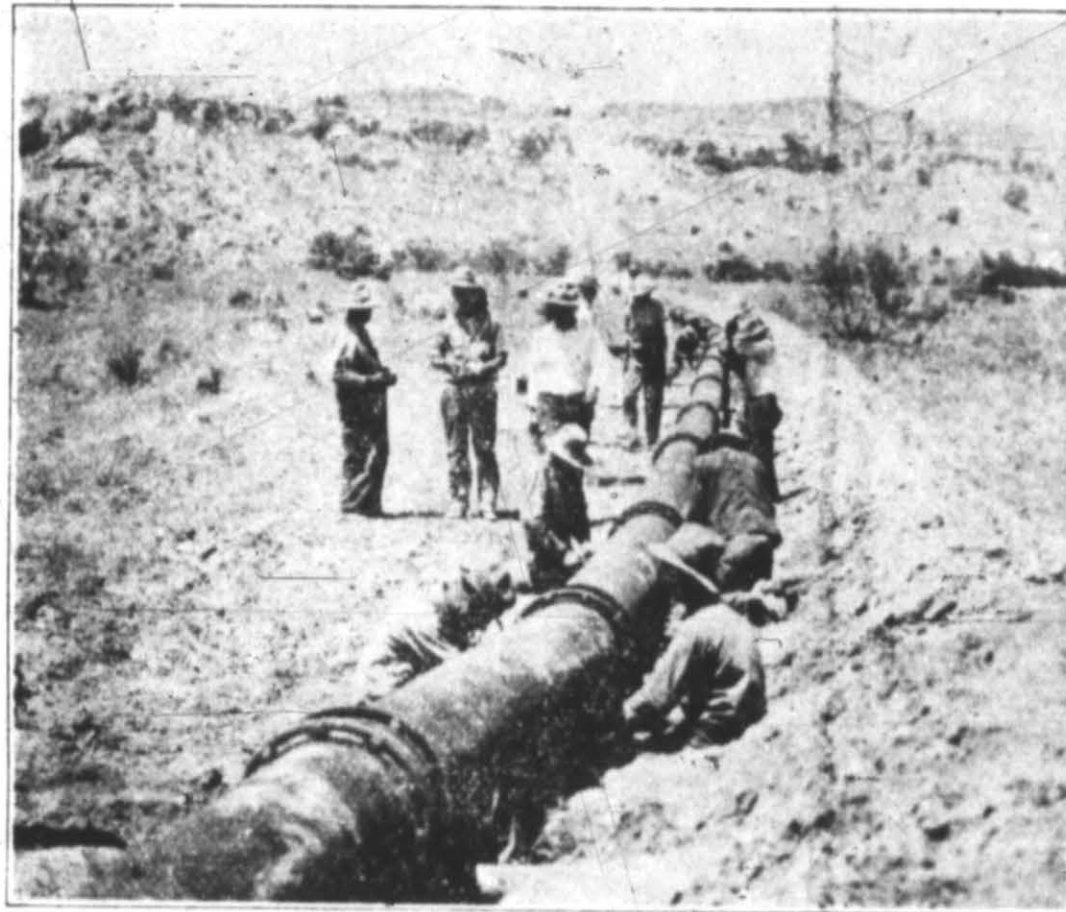
Big Gas Main Which Serves Hereford Crossing Palo Duro Canyon
