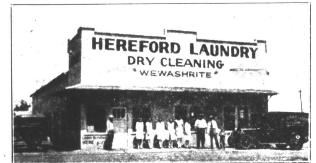
The Hereford Laundry Plant and Group of Employees.
