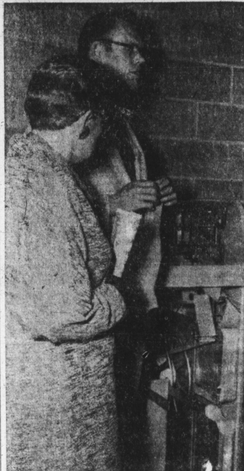
THOROUGHLY EXPLAINED—Ray Bosley, Southwestern Bell Telephone plant employee, explains the long distance recording machine to one of the many crowds that toured the plant during its open house last week. A complicated machine, it punches on a tape the time the call was placed, the number from which the call originates, its destination and the time the call ends. The tape is later sent to St. Louis where it is put on another machine, and cards are printed for billing. (Staff Photo)
