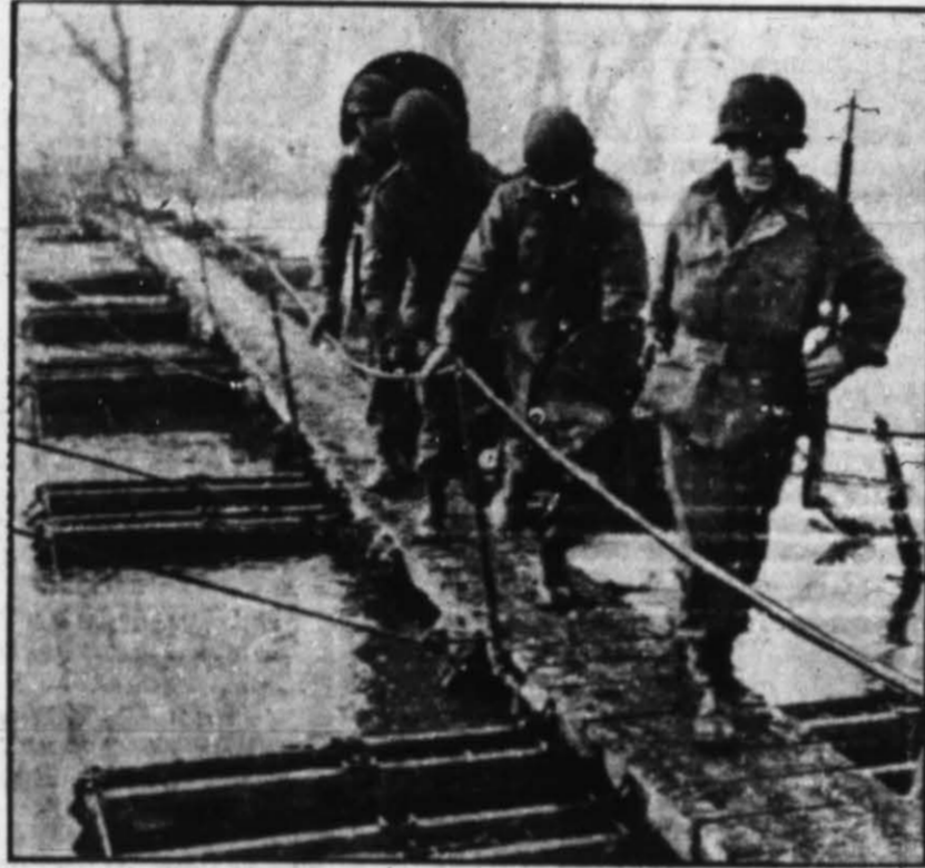
In the new Western Front offensive, a U. S. 9th Army wire team carries drums of communications wire over a pontoon foot bridge across Roer River in Germany. (Signal Corps Radio-Telephoto.)
