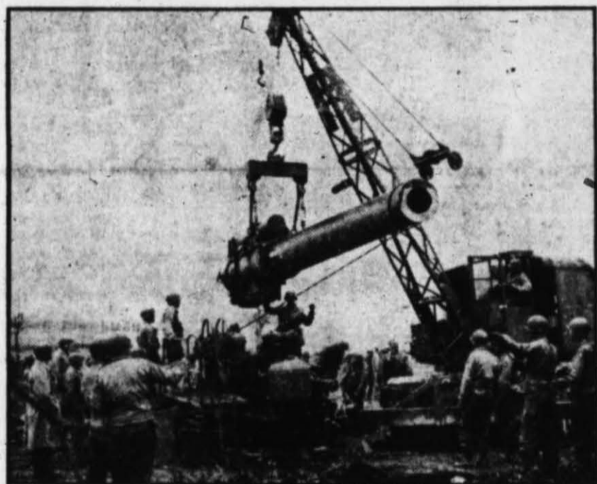
Here you see the same piece being craned onto its mount under supervision of Army engineers. (Signal Corps photo.)
