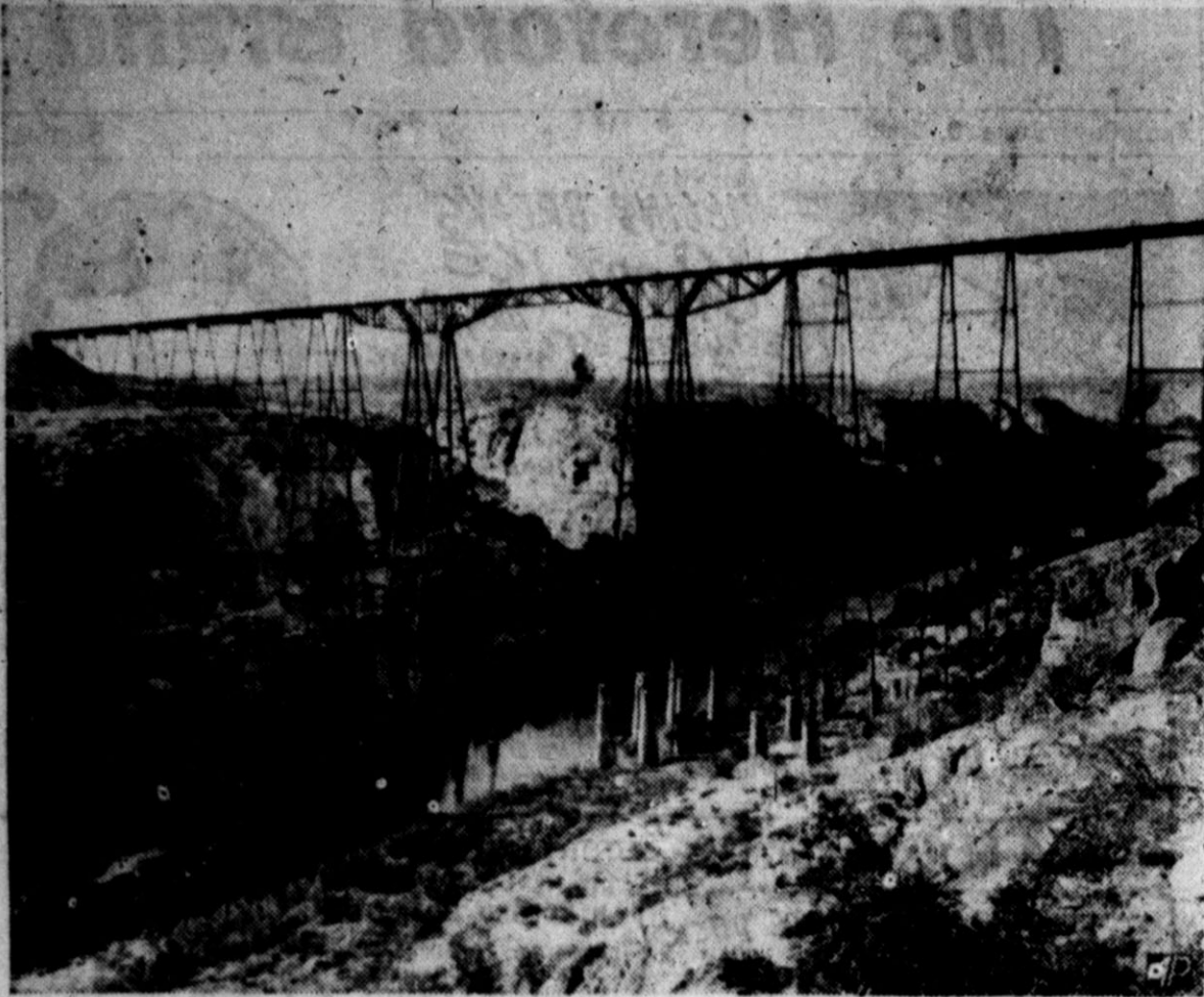
This is the 8-year-old bridge of the Southern Pacific Railroad across the Pecos River gorge near Langtry, Texas. It is now being dismantled for probable reassembly at Guatemala City, Guatemala. The bridge, which is 321 feet high, is said to be the highest such bridge in the United States and the fourth highest in the world. (AP Photo).
