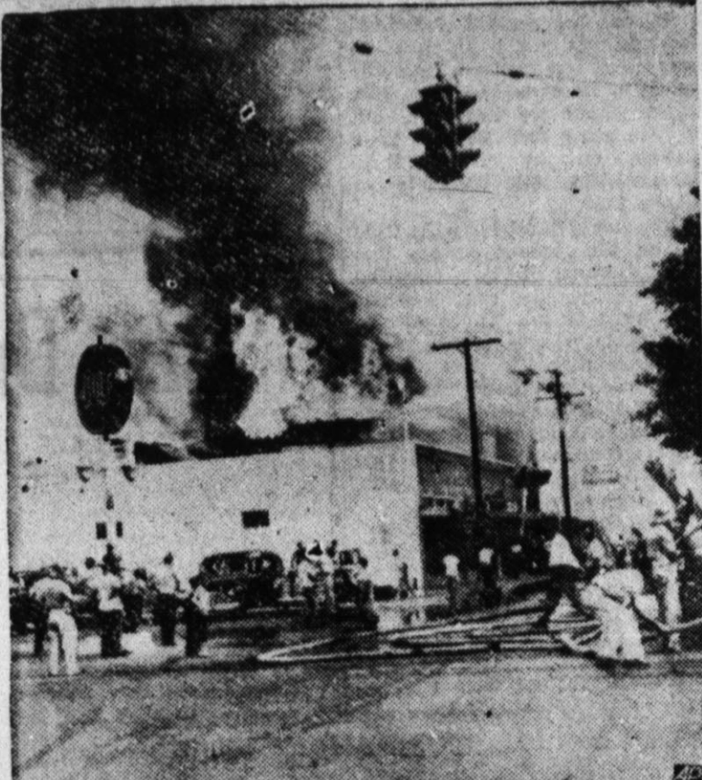
ORANGE BUSINESS BUILDING BURNS —Smoke and flame pour from the top of one of three business buildings that burned in the Orange, Tex. business district, August 12. Shortly after this picture was made the wall of the building collapsed. (AP Wirephoto)
