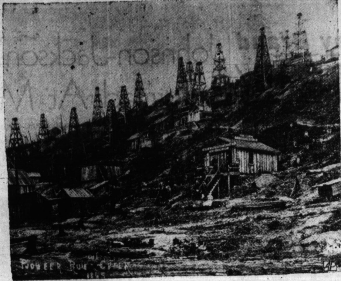
HILLSIDE OIL DERRICK SCENE 83 YEARS AGE —The discovery of oil at Titusville, Pa. by Edwin L. Drake on Aug. 27, 1858 started a wild oil rush and an industry that is currently celebrating its 90th birthday. Derricks seemed to spring up overnight everywhere. Typical of these booming days is this scene of a hillside, overlooking Pioneer Run in 1866. Scenes like this belong to history, however, since the modern oil industry spaces its wells as an established conservation practice. (AP Photo)
