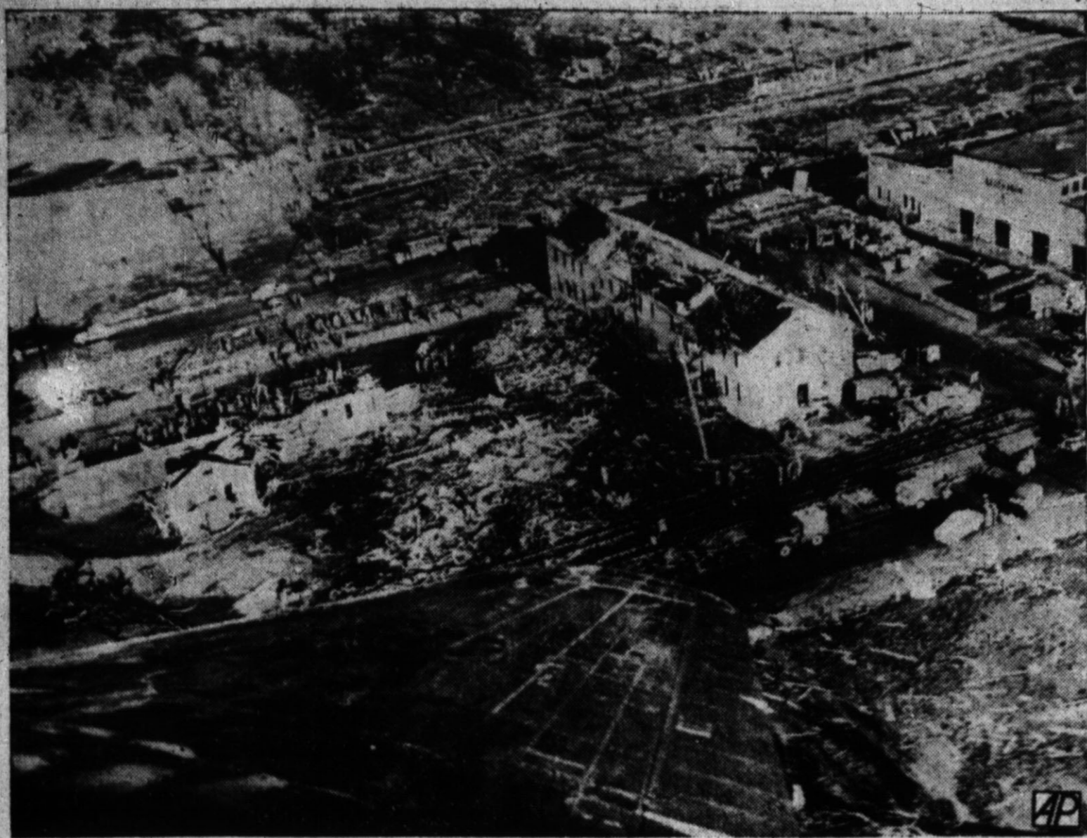
TORNADO LASHED AIR BASE—This is the wreckage of two barracks and a mess hall at Slack Air Force Base which was struck by one of the series of tornadoes that bounced through East Texas, western Louisiana and southern Arkansas Sunday (Feb. 12). Five airmen and a civilian were killed at the air base. One barracks (center) was leveled and the other (right) battered. The wrecked mess hall is at the left. (AP Photo)
