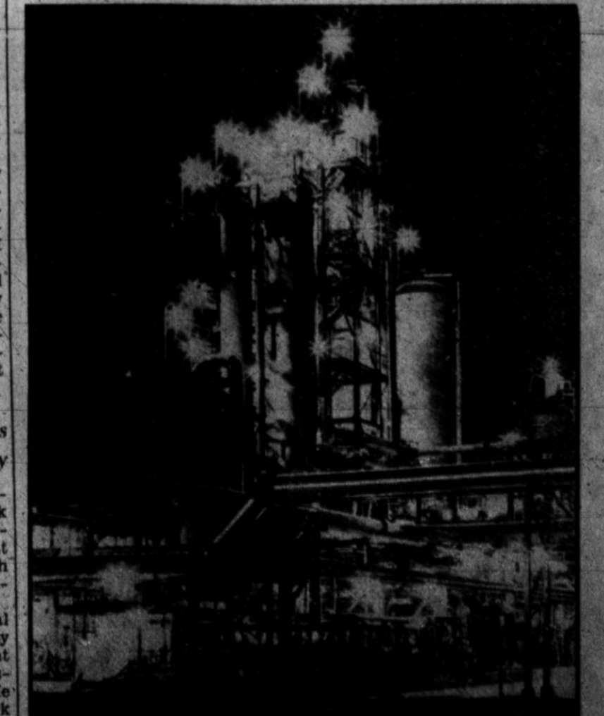
IT'S TEXAS, NOT TIMES SQUARE —The lights of a new lubricant refinery at Beaumont, Tex., blaze in the night. These bright lamps are in the plant's phenol unit where petroleum is treated to free high-quality oils by dissolving low-quality oil.
