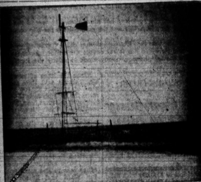
MOST EXPENSIVE WELL IN COUNTY —This well on the A. L. Cross place is said to be the most expensive in Deaf Smith County. The county drilled twice in an effort to get as good a well as Cross said he had before they moved the well out of Harrison Highway right-of-way. The county finally settled by paying him for a third well, making the final cost total $600.
