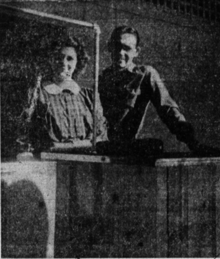
THE COMMUNITY CLEANERS is owned and operated by Mr. and Mrs. Gwynn Owens, who are shown above standing behind the counter at the new establishment in Park Avenue Village. The pipe shown in the picture is a rack for holding clothes while the clerks are making change. The couple formerly operated a cleaning business in Hale Center. —Grand Staff Photo
