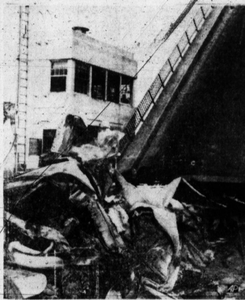
This is the wreckage of a car that smashed into the raised Galveston Causeway drawbridge and burst into flames. Ralph E. Murphy, 29, of Lamarque, the driver, was killed. The drawbridge was put out of service and hundreds of cars had to be rerouted over the old two-lane causeway. AP Photo
