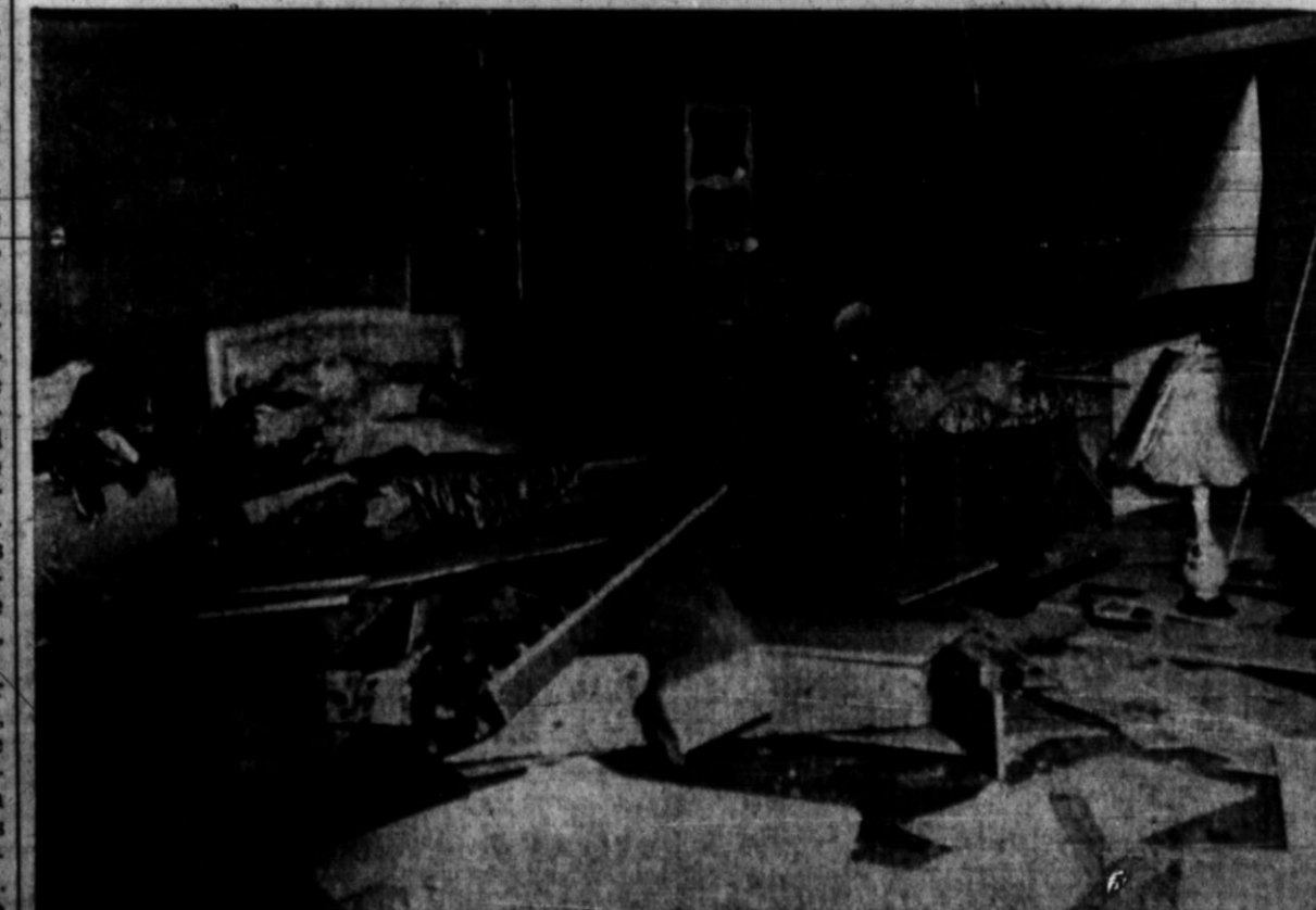
THE HIGHEST PERCENTAGE of loss from Monday's blast was suffered by the Home Beautiful Decorators shop owned by Mrs. Ray Cowser. About 90% of the stock was destroyed by the blast, which took its full force through the wall separating the Washateria and the decorator shop. Alex Thompson Photo
