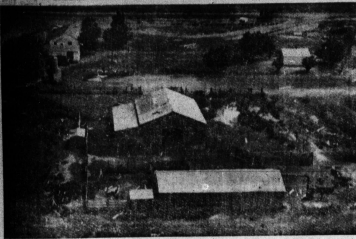
THERE WERE NO identifications given for the Mystery Farm shown above. The first city and the first rural reader to make the correct identification will receive two theater tickets. The second person in each group to identify the place will be given a free wrestling ticket. —Brand Staff Photos.
