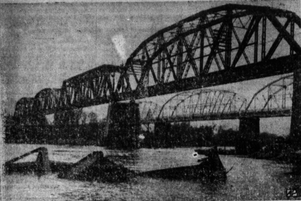
SCRAP FOR DEFENSE—Portions of the collapsed Katy railroad bridge near Denison are to be salvaged from the Red River to furnish scrap for the national defense drive. Visible in the foreground are portions of the old bridge that washed out in a flood of 1908. Some old coal cars had been moved onto the bridge to try to hold it. The cars, too, will be salvaged.—AP Photo.
