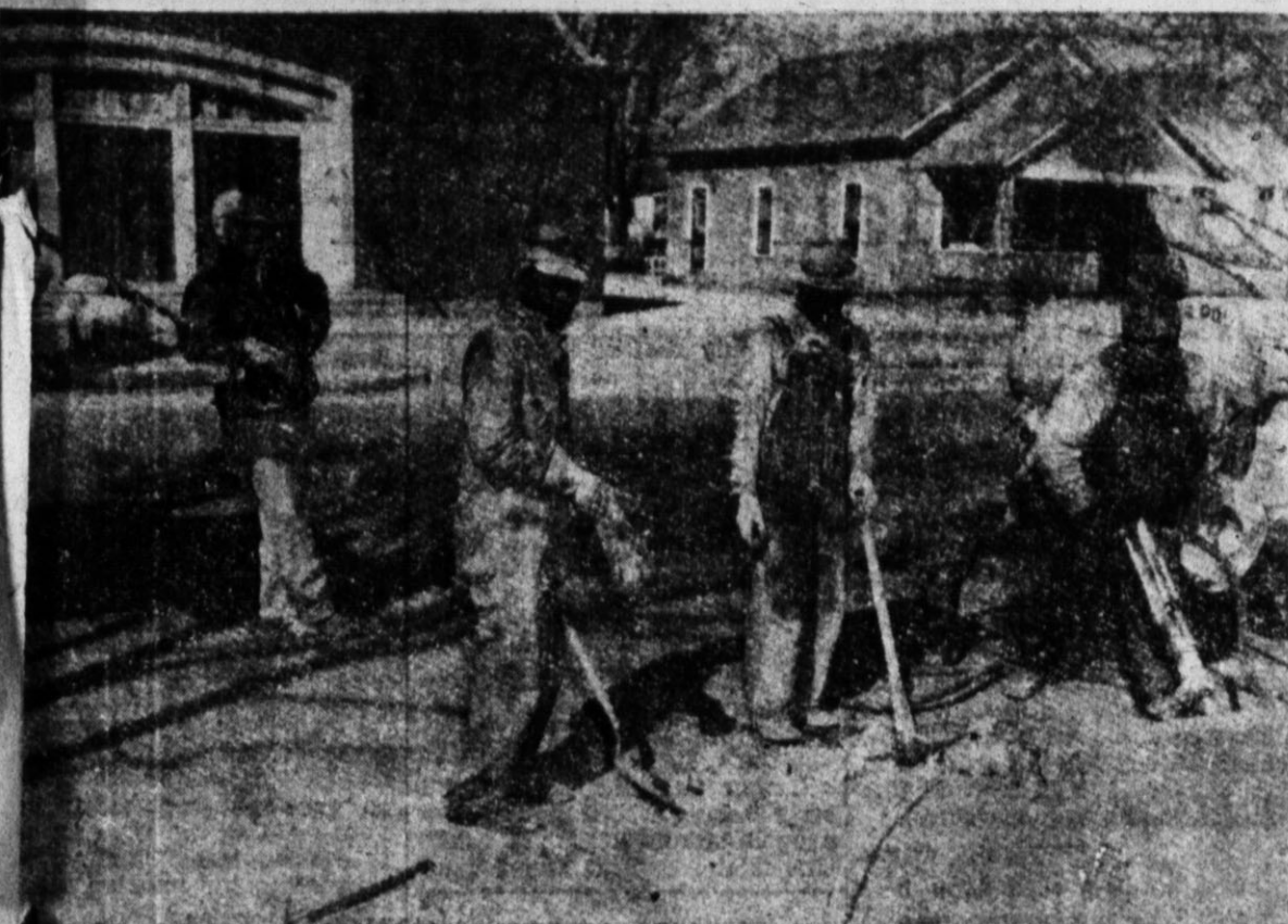
KERR AND MIDDLETON workmen are shown above pounding the curbing to pieces with an air hammer in front of the First Baptist Church before they widen Main street north. —Brand Staff Photo.
