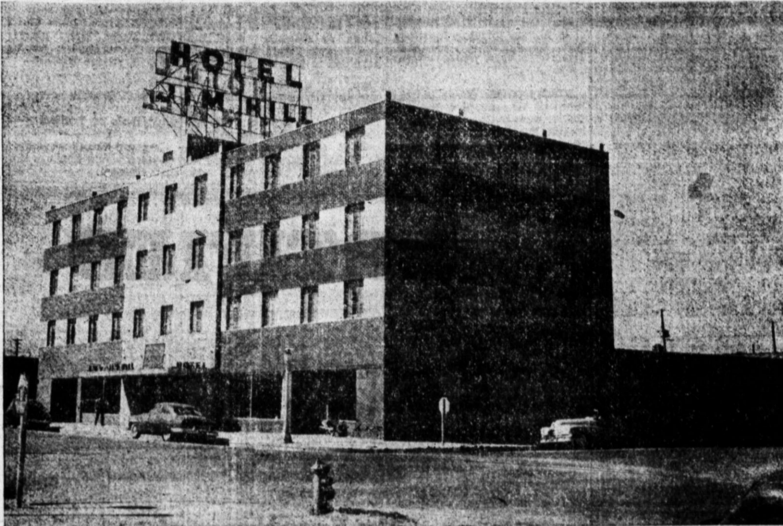
HOTEL JIM HILL, headquarters for the 1951 District 2T-1 Lions Convention in Hereford April 29-30 and May 1. The hotel is located in the center of town on Third Street, one block east from Main. All of the convention meals will be served here, except the Ladies Breakfast Monday morning. Visitors will also register at the hotel for hospitality books.
