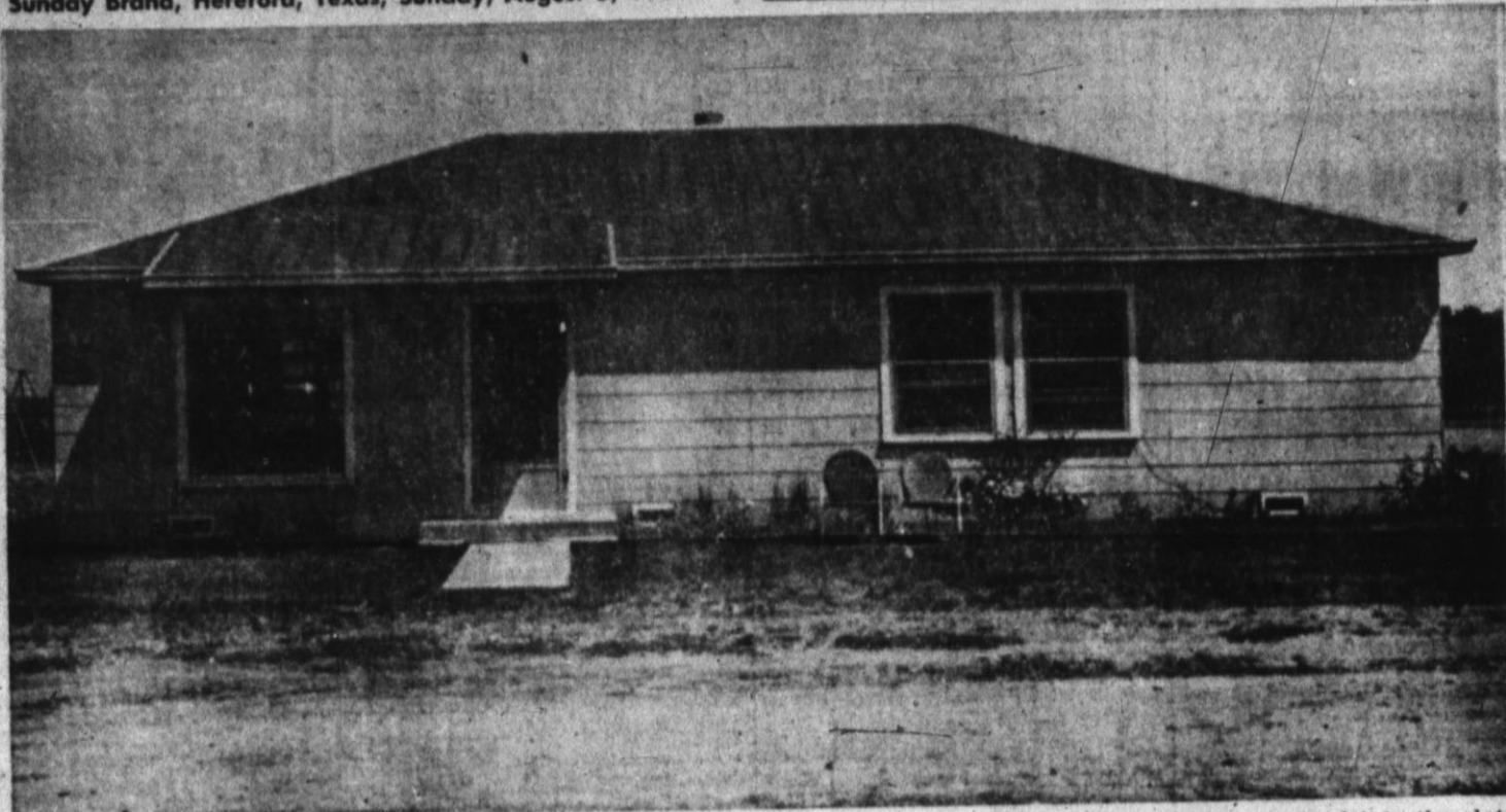
TYPICAL OF THE SMALLER new homes in Friona is the Roy Wilson residence, shown above. Wilsons moved into the slate-sided house on June 26. The Wilsons have one daughter, Lynn, age five. —Brand Staff Photo.
