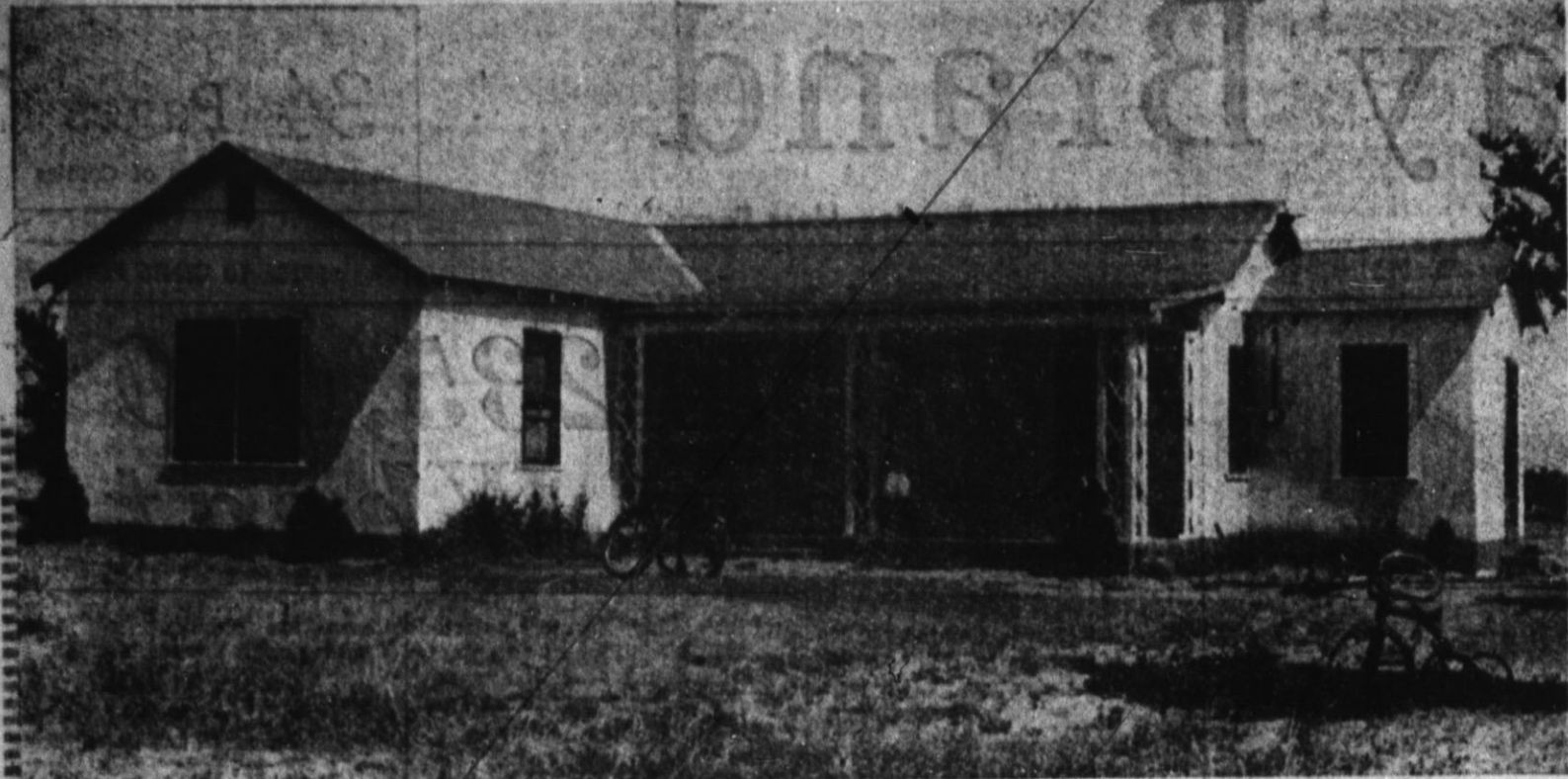
THE MAYO PHIPPS home started with the two rooms at the left and was completed during the past year. The Phipps have one son, Dewain, who is in the first grade at Central school.—Mrs. Merlin Kaul Photo.
