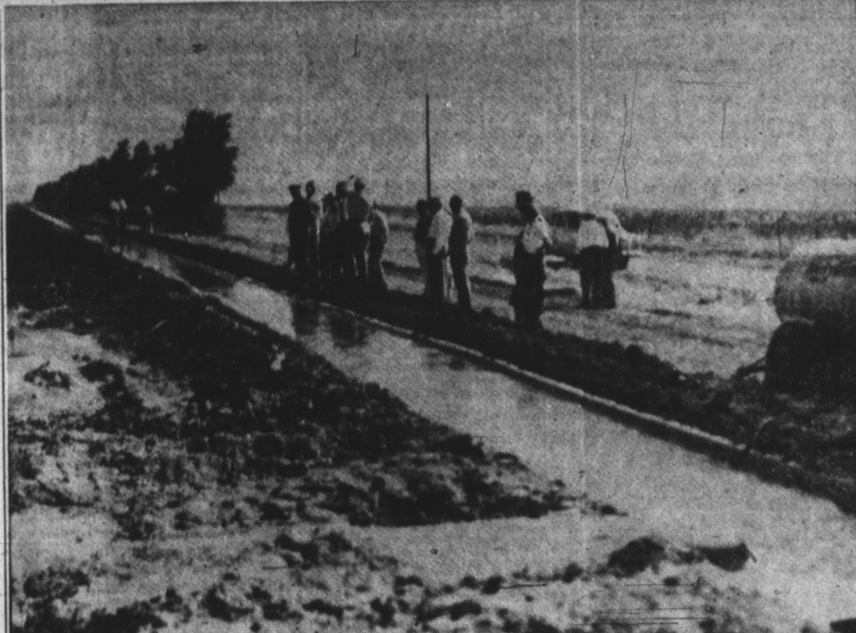
CONCRETE DITCHING on the Anderson farm near Hereford was one of the sights of inspections and discussion on the farm tour last Tuesday and Wednesday as a climax to the irrigation short course held here.
