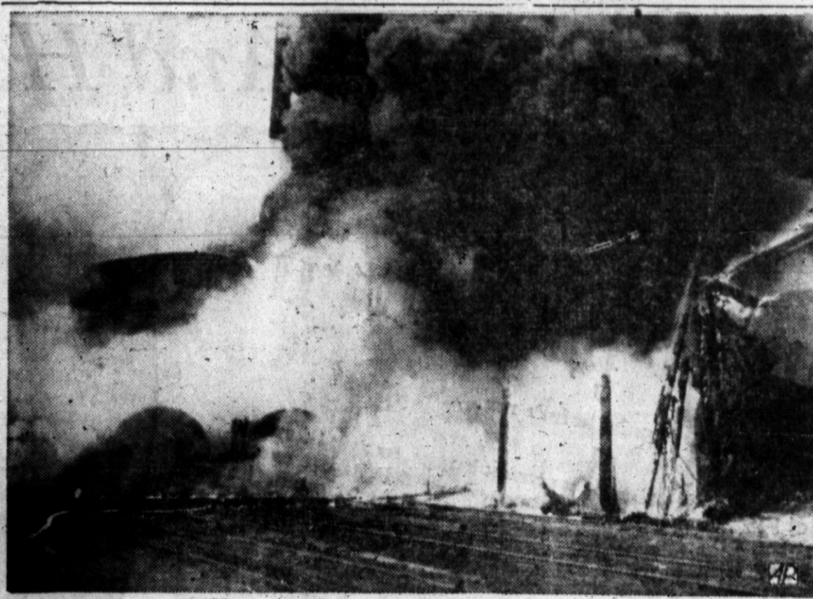
CREOSOTE FEEDS MILLION DOLLAR BLAZE NEAR TEXARKANA -- Damage estimated at $1,000,000 at the $2,000,000 International Creosoting and Construction Company plant near Texarkana resulted from a fire which broke out early on the morning of April 2 and was still smoldering 30 hours
