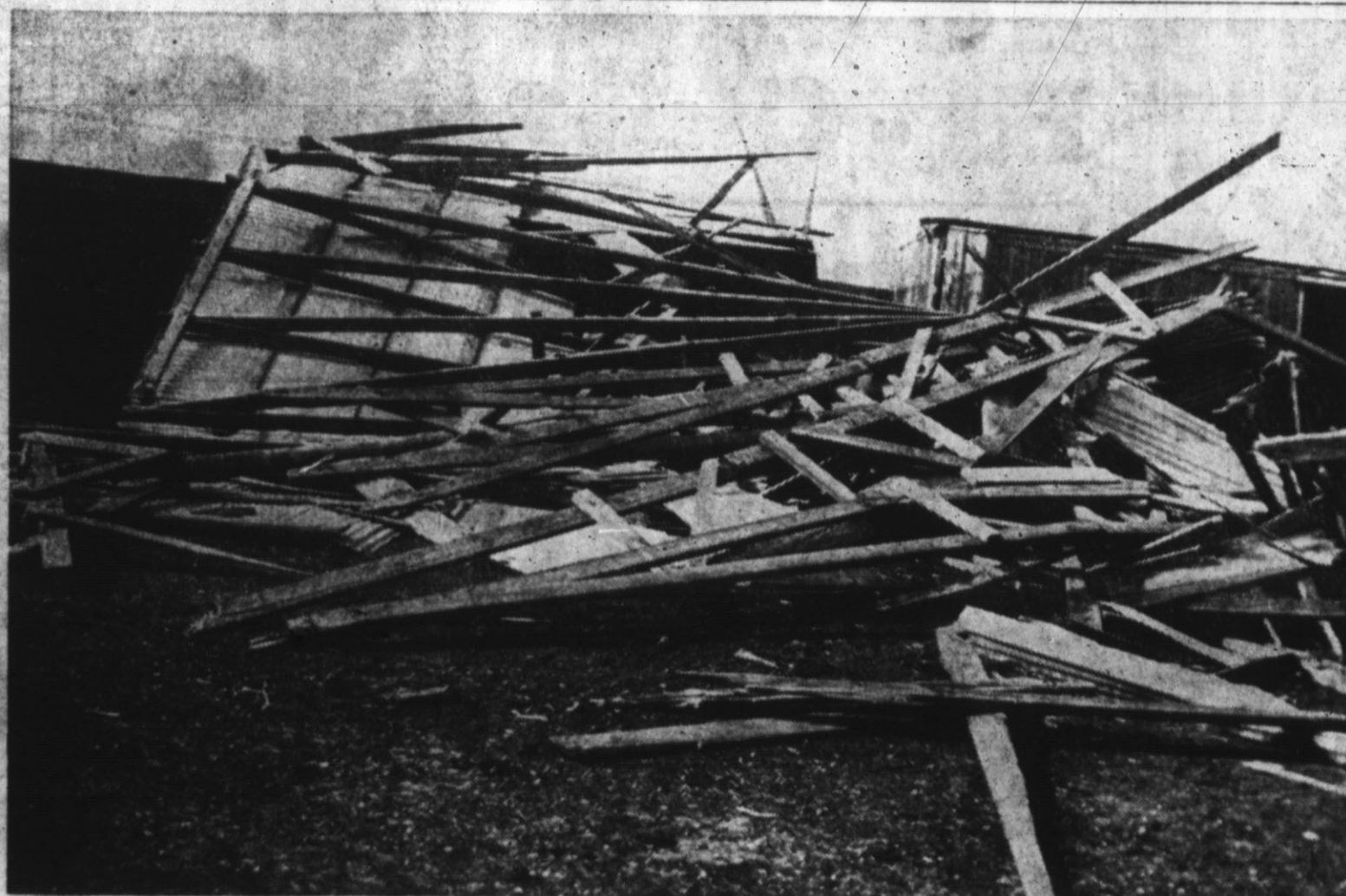
A BIT OF FREAK WIND lifted a shed on the Malone Dairy, about two miles southeast of Hereford, Tuesday afternoon and dropped the whole thing into a nearby pig pen, killing one porker and injuring three others. The accident occurred about 4:15 o'clock, shortly after Hereford had received a sprinkle of rain. It was not known whether the damage was done simply by high wind or from a small twister. There was no other wind damage reported in the county. (Staff Photo)
