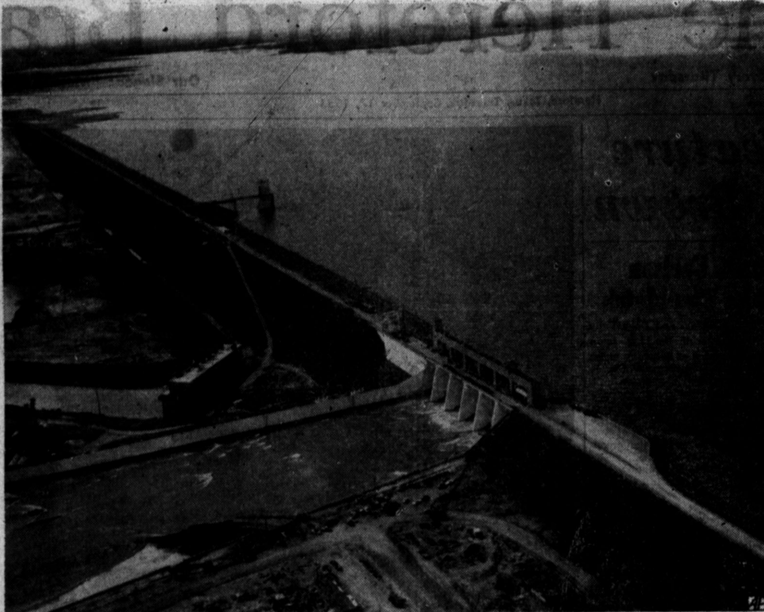
FALCON DAM -- This air view of the Falcon Dam and spillway was taken from a point downstream from the dam on the American side and looking toward the Mexican side of
