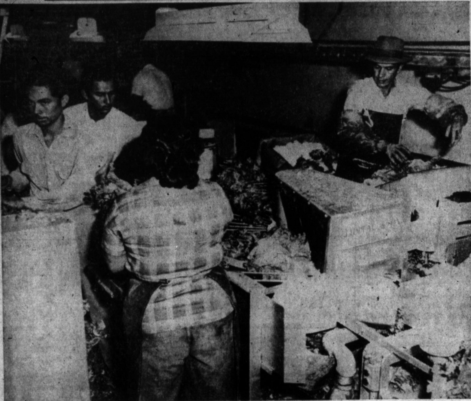
LETTUCE PACKING, which combines as much machinery as possible with hand labor, has been rolling along at the Chas. Huston sheds west of Hereford, but may be slowed down considerably by Friday afternoon's hail storm. The lettuce is brought into the sheds in special carts, each head is checked, left, then put on a turntable which carries it to the packer, who packs two crates of lettuce almost at the same
