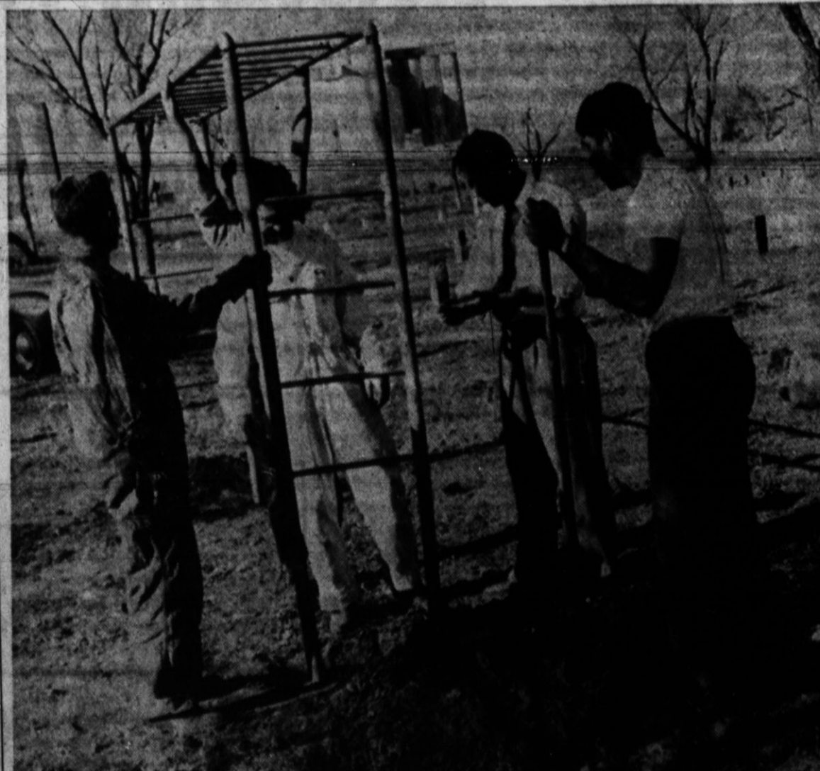
TWO PIECES OF PLAYGROUND equipment donated by Mrs. James W. Witherspoon were installed by members of the Hereford Junior Chamber of Commerce in Joyce Park Sunday afternoon. Those installed are the overhead bars, shown here, and a slide. Kenny Gear is constructing a swing and a see-saw, which are being partially paid for with funds the Jaycee-ettes had raised for the project. Working on the project Sunday were, from left: Don Fudge, Bill Howard, Dennis Lomas, who is almost hidden behind Howard; Gerald Kirkland, and Sam G. Nelson. (Staff Photo.)
