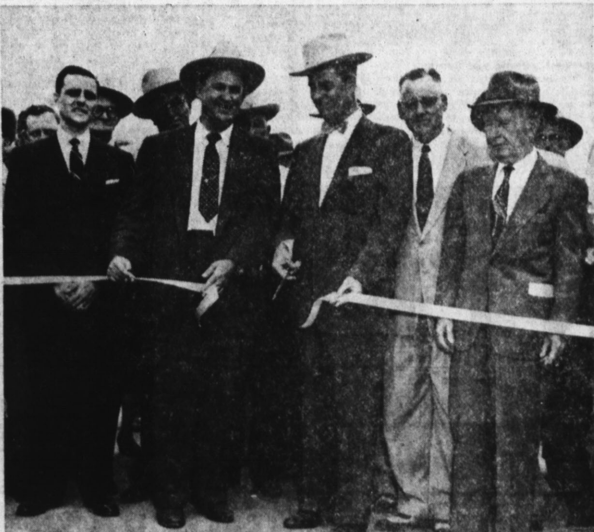
CHAIRMAN OF TEXAS Highway Commission E. H. Thornton, Jr., is seen with the scissors which snapped the ribbon Sunday afternoon to officially open the new Canadian River Bridge, near Tascosa. In the picture, left to right, are: Kim McAbee, Dalhart, president of the Texas Highway 51 Association, Marshall Formby, Plainview, Texas Highway Commissioner, Mr. Thornton, Julius W. Cox, Boise City, member of Oklahoma Highway Commission, and Robert J. Potts, Harlingen, Texas Highway Commission.
