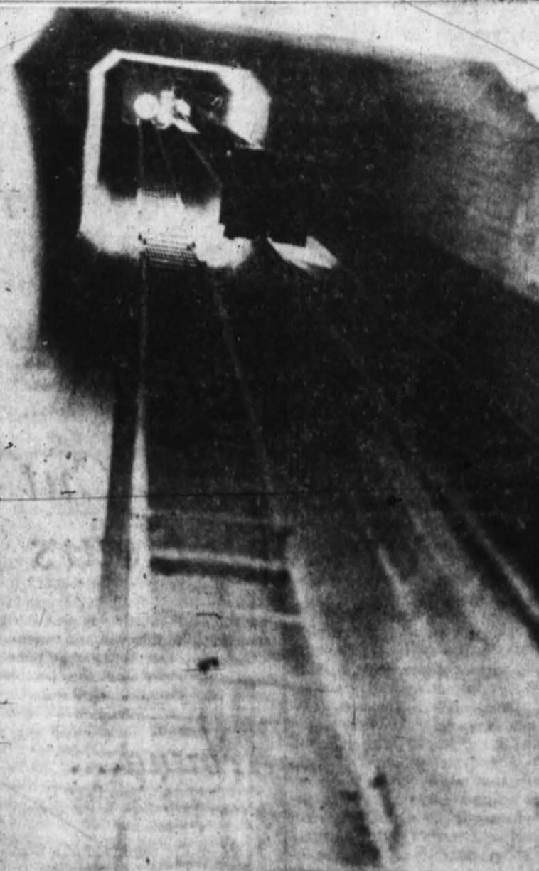
ACCIDENT SCENE, above, shows the 147-foot, 10-inch ladder down which one workman lost his life Wednesday, and a second, 30 feet down the ladder, was almost knocked loose when struck by the falling body.
