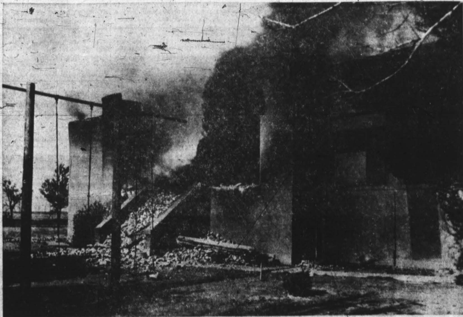
SUMMERFIELD SCHOOL HOUSE, used as a community meeting place since Summerfield was consolidated with the Hereford school system, was a total loss when it caught fire and burned Saturday morning.
