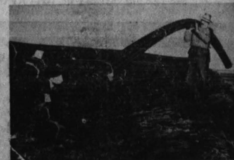
Plastic welded joints assure years of trouble free service. Every CARLON Gas Line is completely pressurized and tested before covering.
