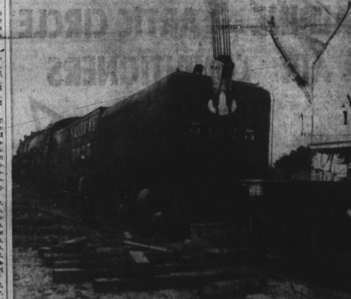
TRAIN TROUBLE -- It took workmen 10 hours to get this locomotive back on the track Thursday after the heavy Santa Fe engine turned a track on a sharp curve and derailed in Hereford. The train backed onto a siding which wasn't meant to be used by such a heavy locomotive, a railroad spokesman said. (Staff Photo)
