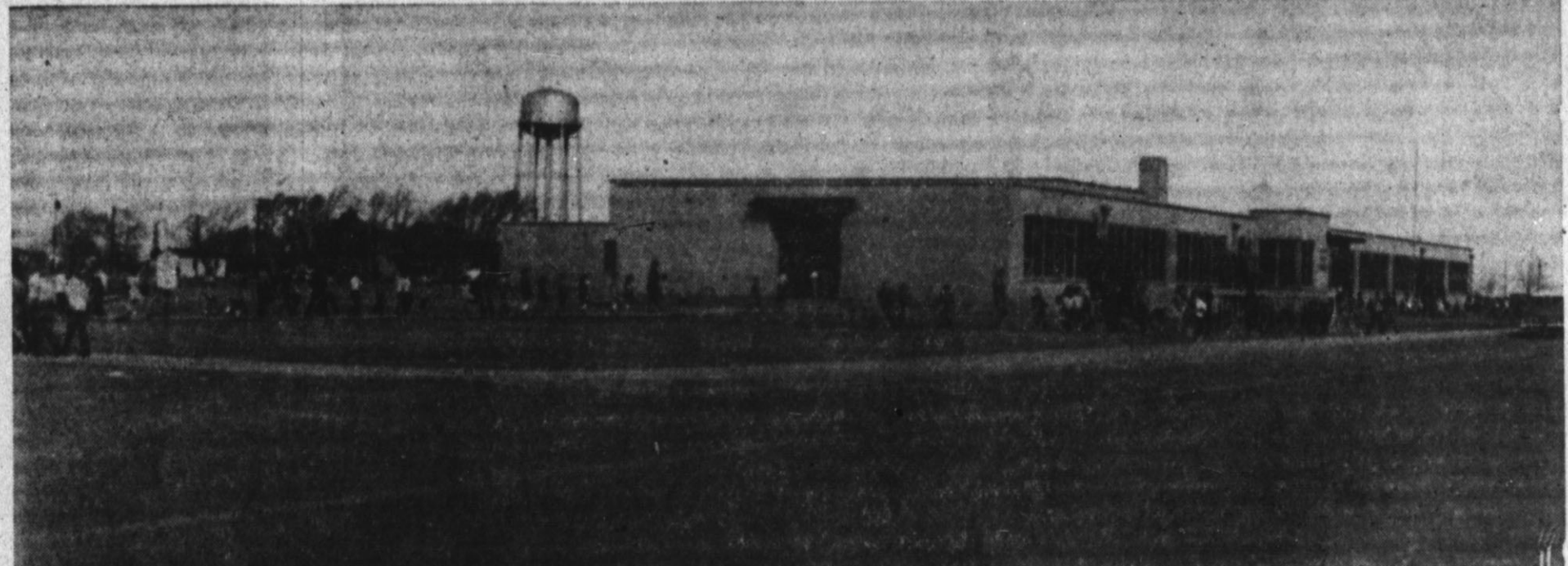
FIRE DRILLS HELD REGULARLY—Regular fire drills are held at all local schools. Here students at Shirley School are returning to class after the all-clear signal had been given. The group in the foreground was led by its teacher to the playground for scheduled activity.
